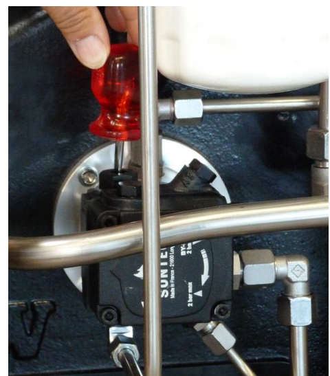
Adjusting the oil pressure
