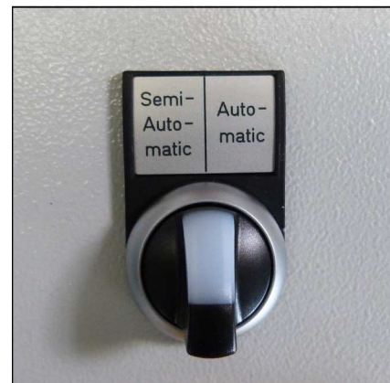
Selector switch auto start function
