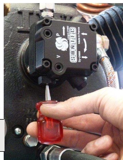
Adjusting the oil pressure
