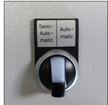
Selector switch auto start function
