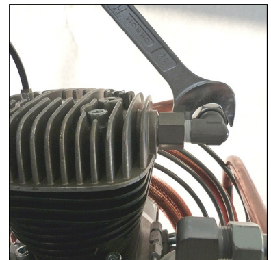
Fig. 6 - Connect pipe connections and tighten
