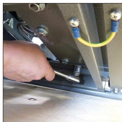
Fig. 2 - Loosen mounting screws of the motor flange
