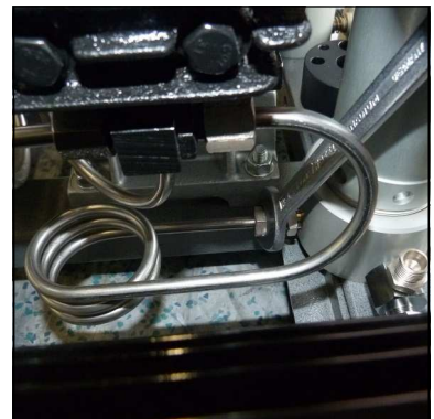
Fig. 2 - Loosen pipe connections of the filter housing
