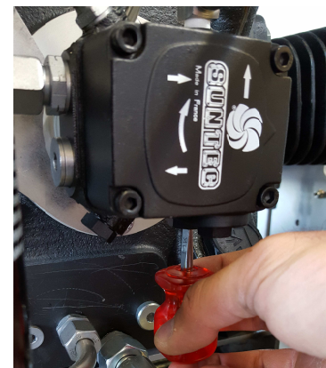
Adjusting the oil pressure
