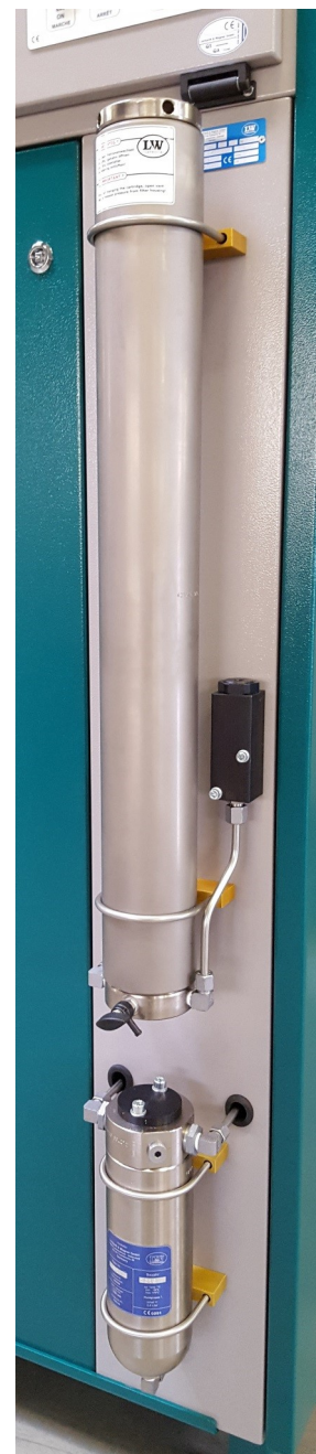
Filterhousing 2.3l (upper), pressure maintaining non return valve and filter unit 0,8l with safety valve (below)(down)
