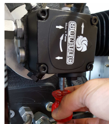
Adjusting the oil pressure
