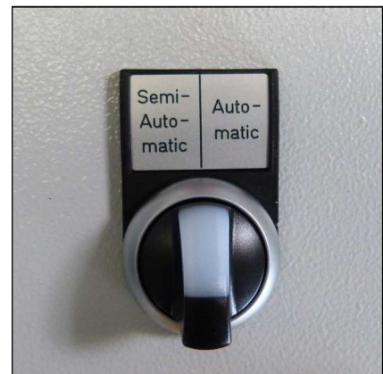
Selector switch auto start function
