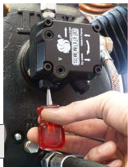
Adjusting the oil pressure
