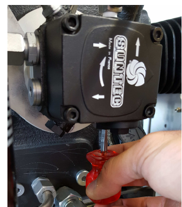
Adjusting the oil pressure
