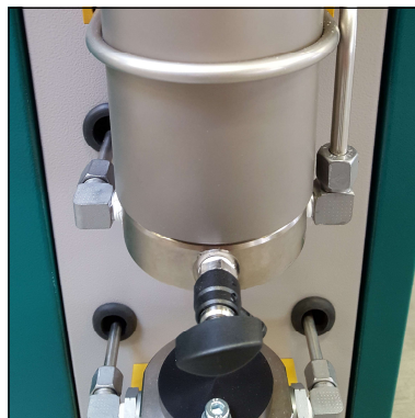
Fig. 3 - Loose pipe connections and nuts
