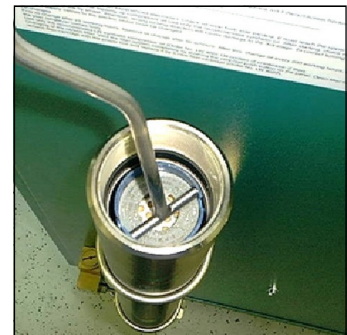
Fig. 3 - Place the T-piece end of the filter key in the top of the filter cartridge.
