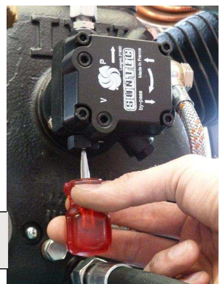
Adjusting the oil pressure
