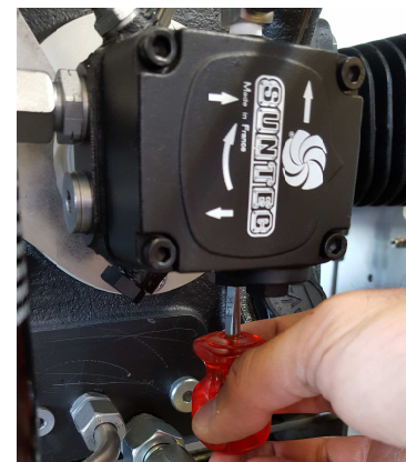
Adjusting the oil pressure
