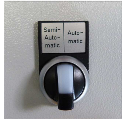
Selector switch auto start function
