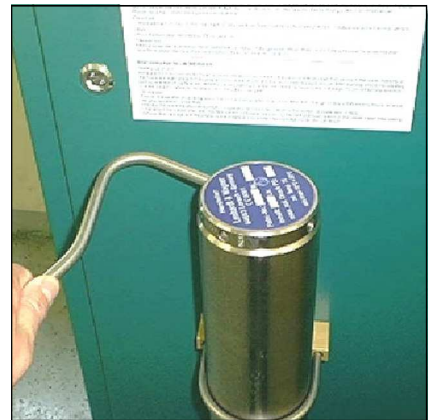
Fig. 1 - Unscrew the filter housing cover.
