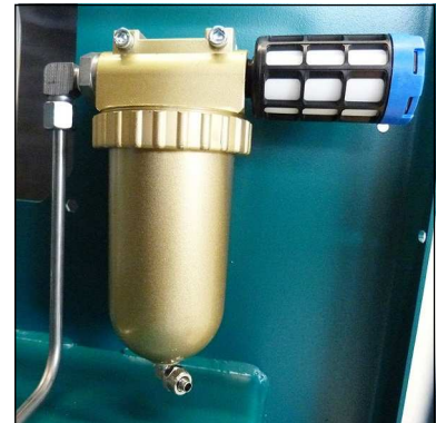
Oil / water separators final stage
