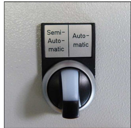
Selector switch auto start function
