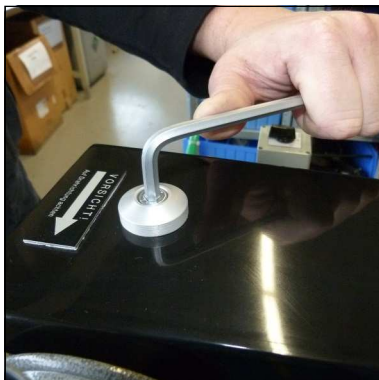
Fig. 1 - Remove top mounting screws
